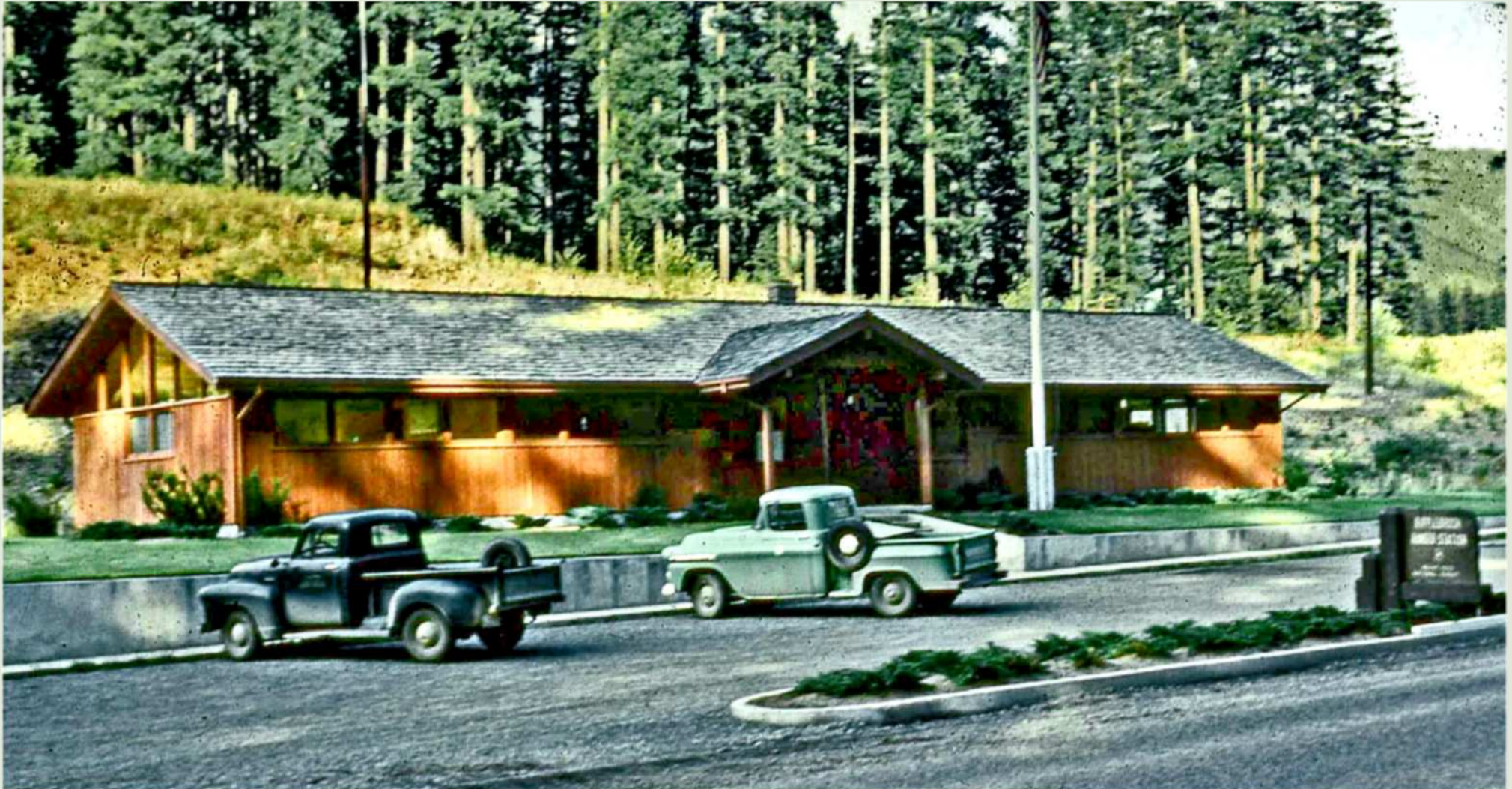
Ripplebrook Ranger Station, Mount Hood National Forest,
