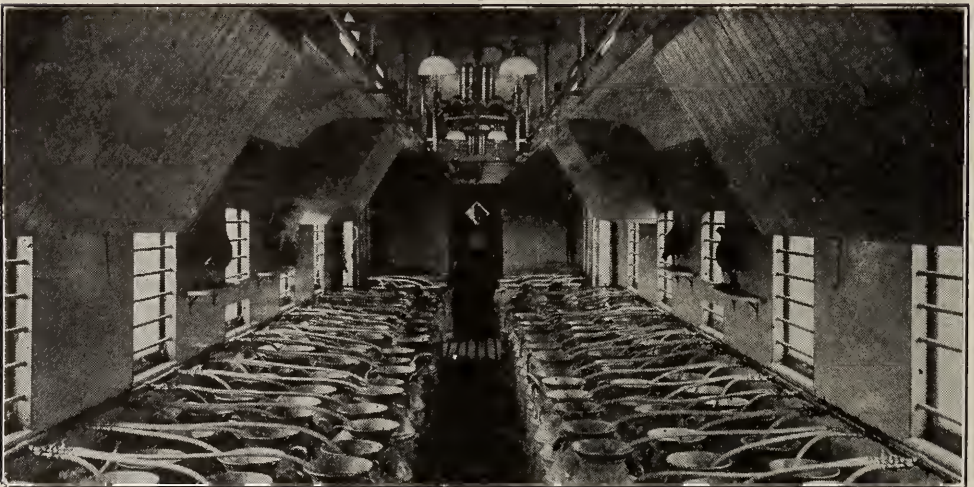
Interior of Fish Distribution Car "Rainbow," carrying One Hundred and Eighty Ten-Gallon Cans, with Air Tubes Attached.
