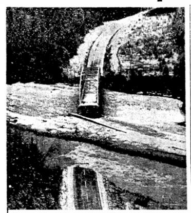
DESTRUCTIVE FORCE of recent flood in Upper Clackamas River area is shown at Carter Bridge site where the swift current has caused a complete change in the channel necessitating a king-sized reconstruction job for the Forest Service. The road shown is the Clackamas River Highway which provides one of the main logging access routes in Mt. Hood National Forest. operators are lucky, that is."
