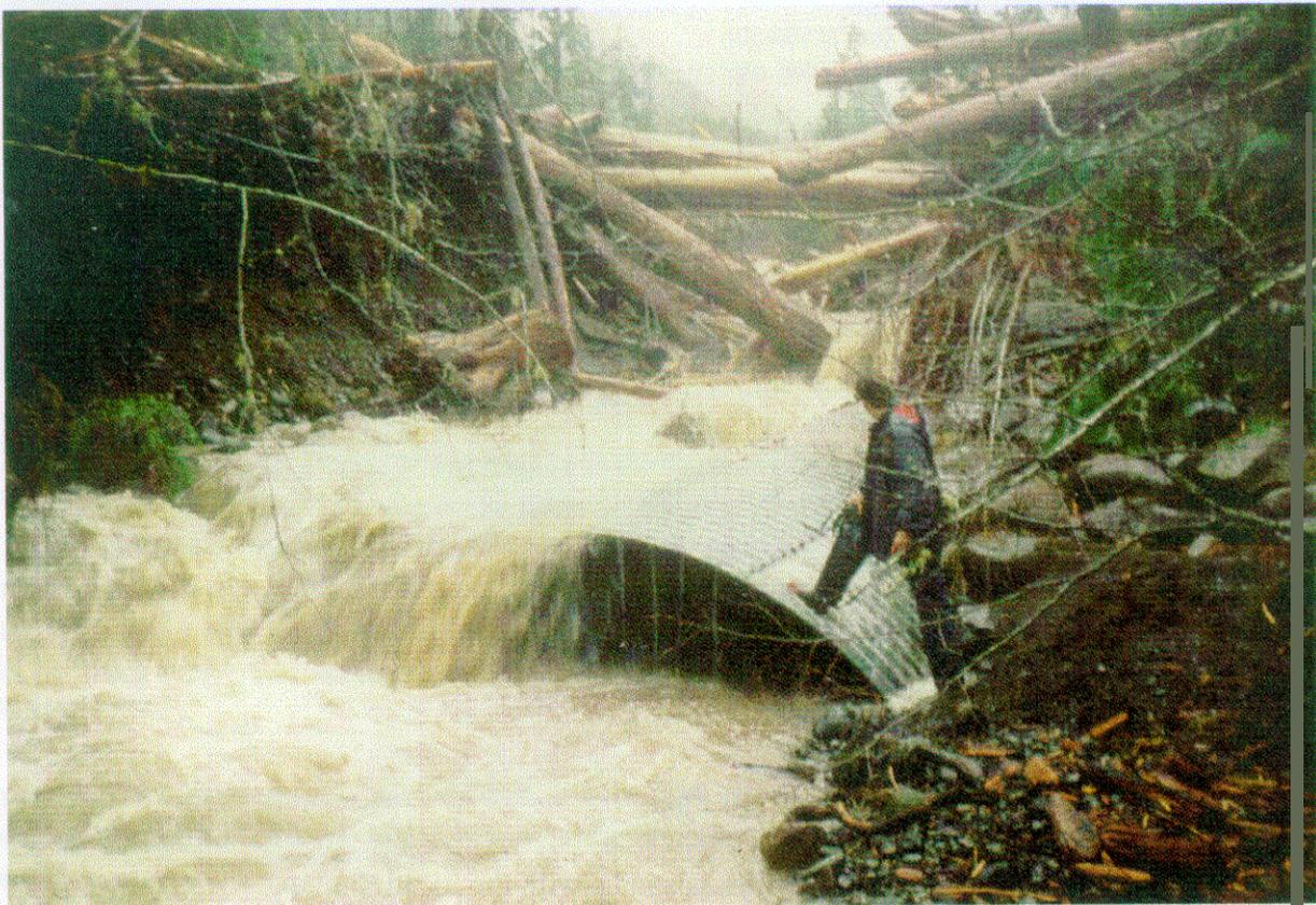
*A three-mile long debris torrent swept through Third Creek, a tributary to Fish Creek, and washed out the main road paralleling Fish Creek during the winter of 1995-96.*
